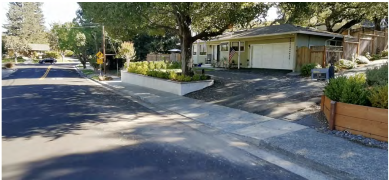
Image 1: Existing sidewalk in front of 246 and 248 Harding Ave
