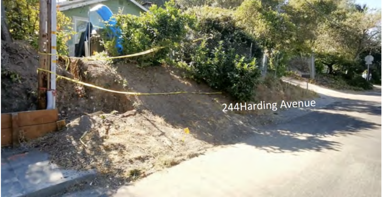
Image 3: Sloped lot and public right of way in front of 244 Harding Ave
