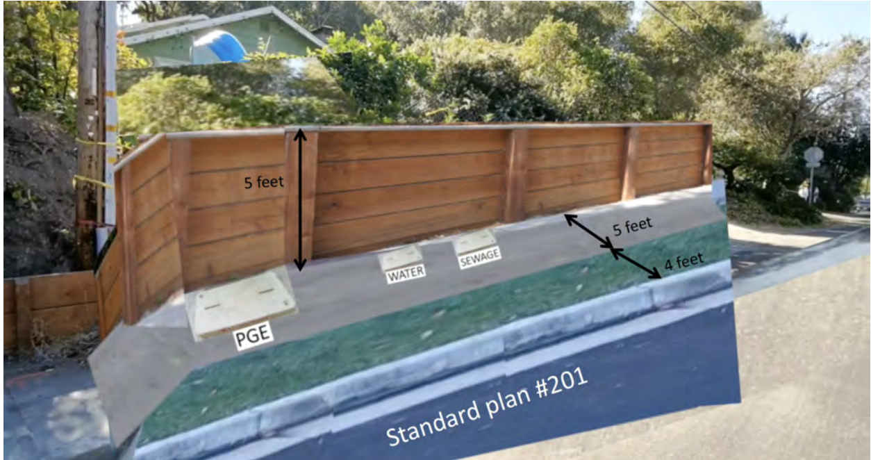
Image 5: Illustrates deployment of standard plan # 201; disregarding the site layout and conditions with a sloped topography.
