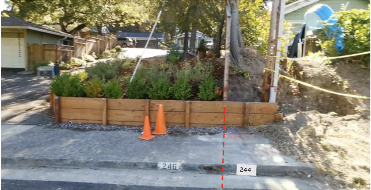
Image 2: Stub sidewalk in front of 244 Harding Ave
